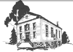
Gates Hall, home to community theatre since 1867.
